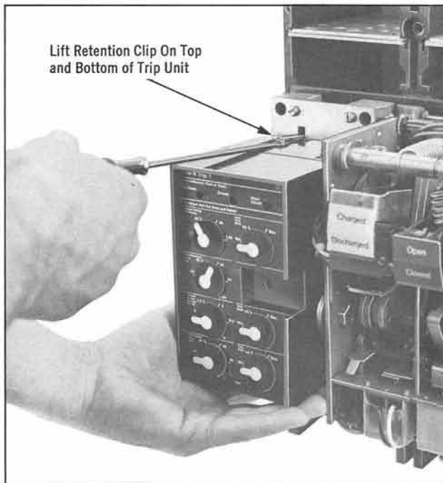
Fig. 39 Removing Trip Unit from Breaker.
