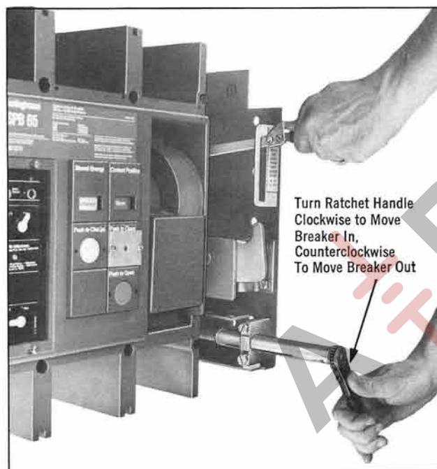
Fig. 19 Operating the Ratchet Handle to Move the Breaker In.
